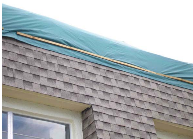
Figure 6. Close up of Fig. 5 showing wooden furring strips securing tarpaulin (from Scheffrahn et al., 2006).
